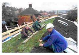
**Fig (3).** In the Hockerton Project (UK, 1996) roofs were covered with soil rather than tiles to increase energy efficiency by trapping heat. The soil acts as a giant radiator.
